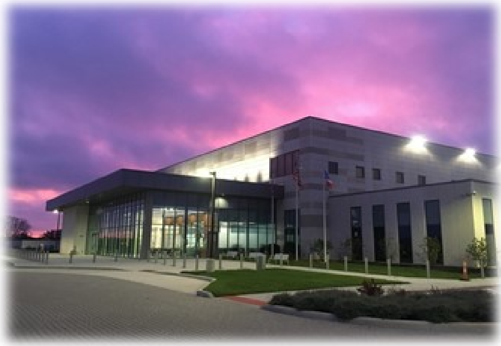
James A. Karnes Correctional Facility Franklin County Sheriff's Office
